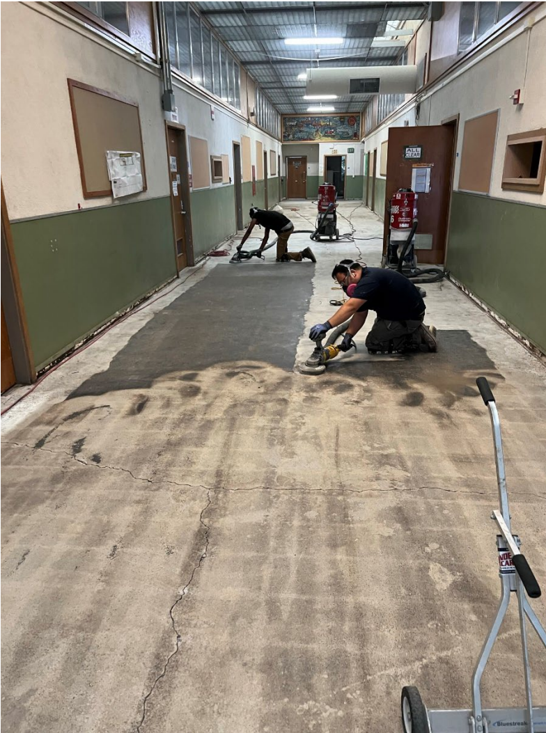
New Hallway Flooring – Floor Preparation and Installation
