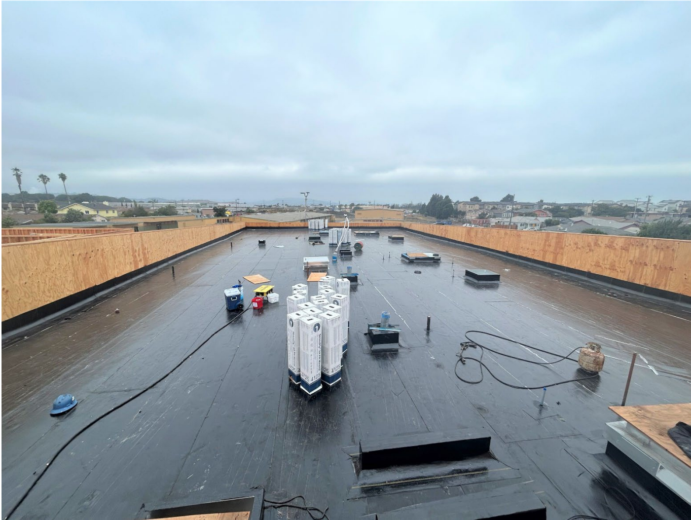
Building A – Roofing Underlayment
