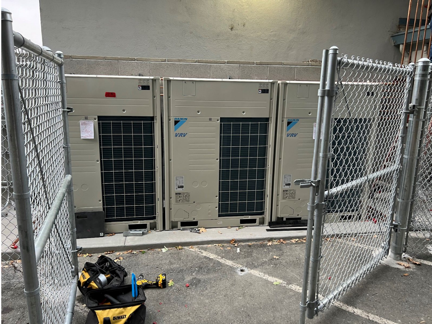
Installation of Condensing Units in Outdoor Equipment Enclosures
