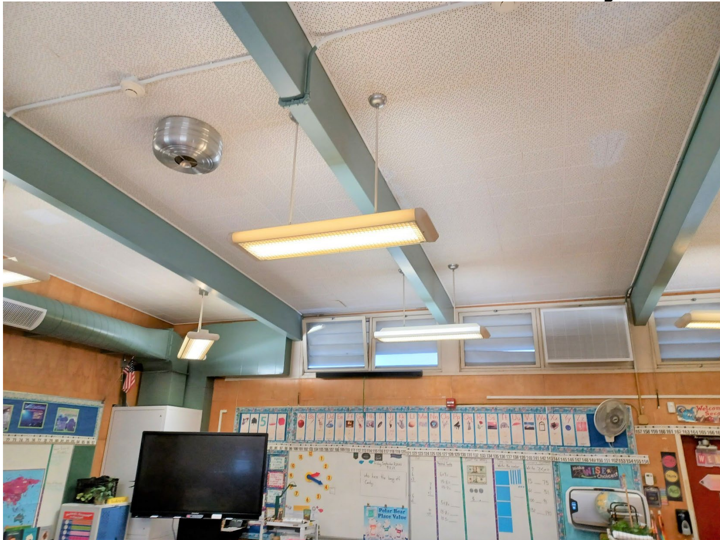
Completed duct work in the classroom
