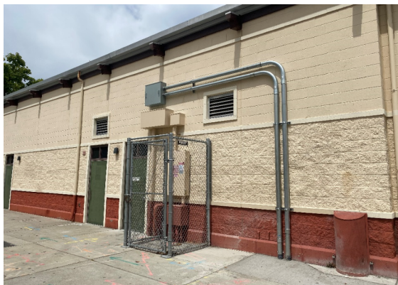
New power conduits at HS electrical room
