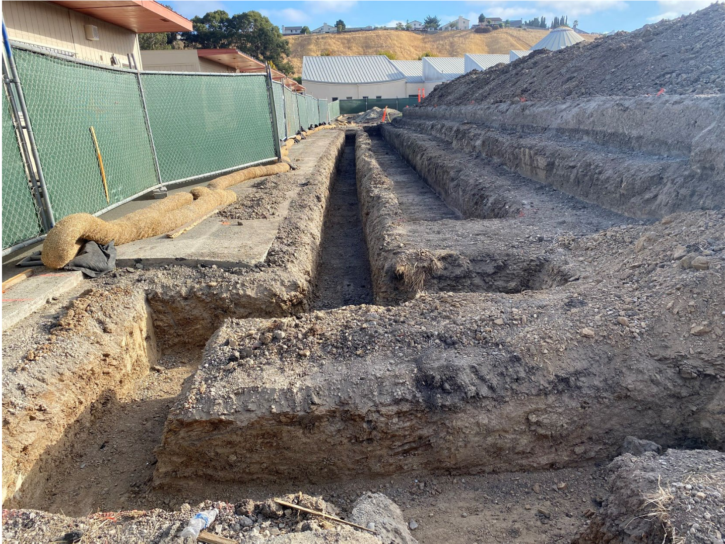
New retaining wall footings excavation in progress
