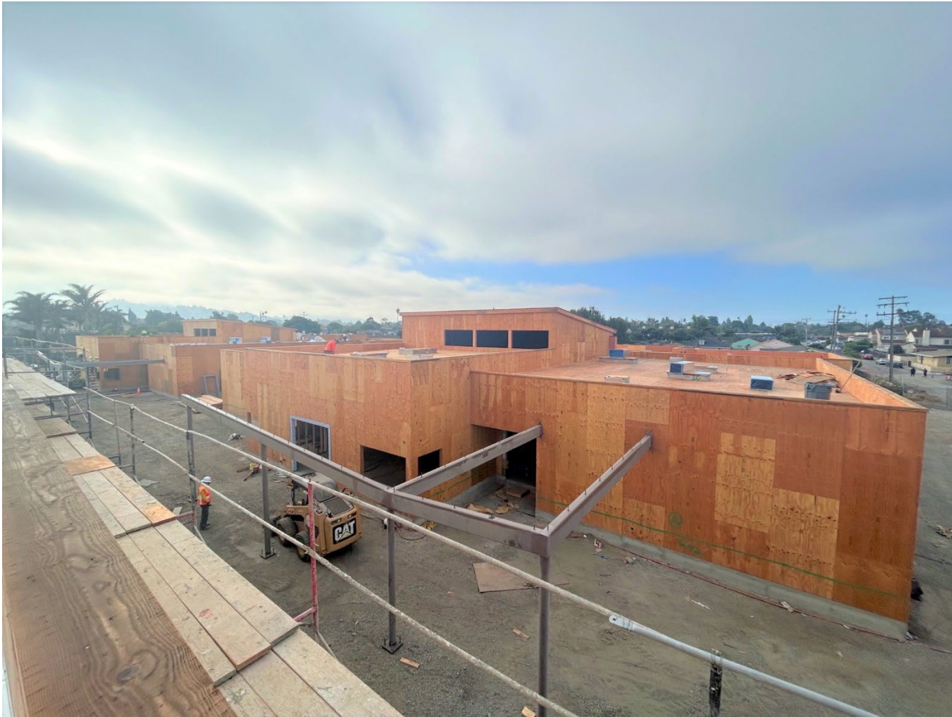
Buildings B and C – Plywood sheathing and awning steel structure installed
