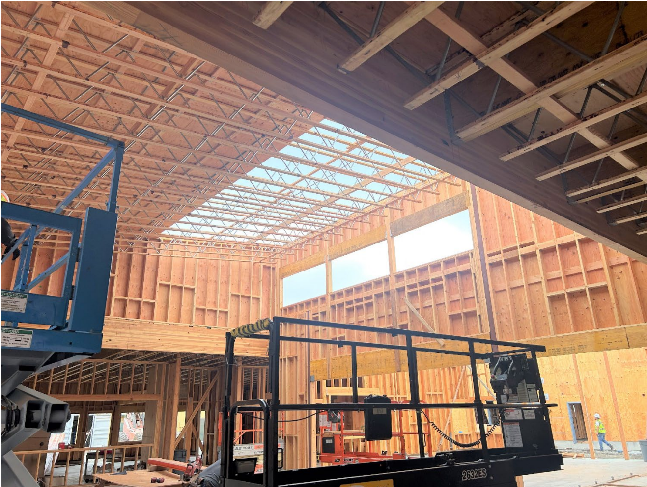
Buildings C Flex Area – Open web joists and sheathing
