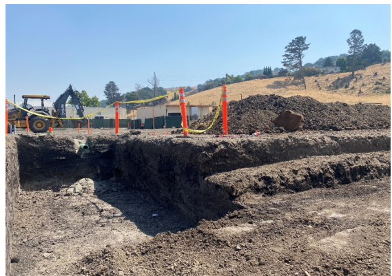
Start retaining wall excavation
