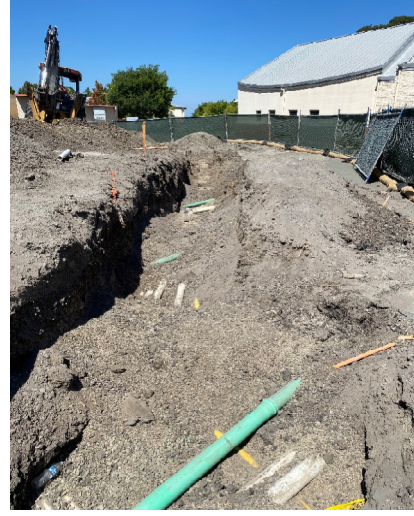
Unforeseen: Expose existing utility lines
